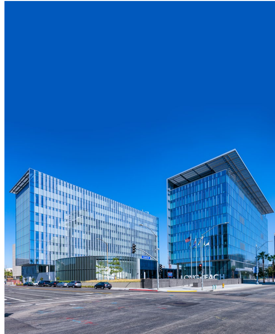
Civic Center - Port of Long Beach Administration Building is on the right.
